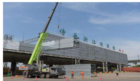
Toll station demolition works commenced at the Zhejiang-Shanghai main line
