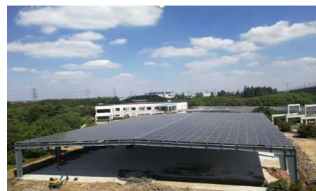
Installation of a distributed photovoltaic power station by Jiaxing Management Office
