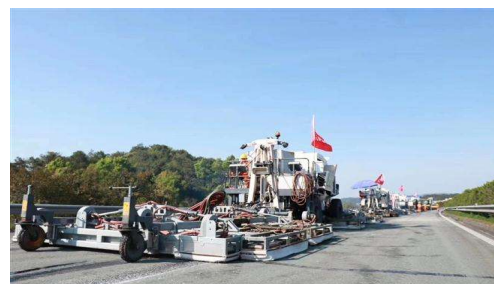
Trial of on-site thermal regeneration technology in the G56 section of Huihang Expressway
